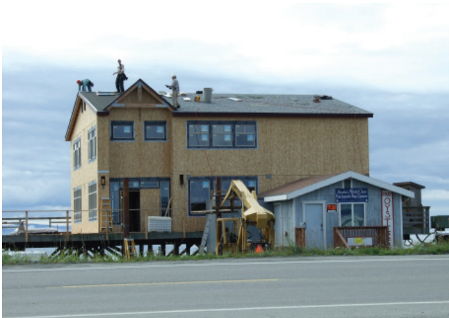
City of Homer planning staff worked successfully to resolve land use issues affecting the construction of a new facility on the Spit to serve as home to the Kachemak Bay Shellfish Growers cooperative.
