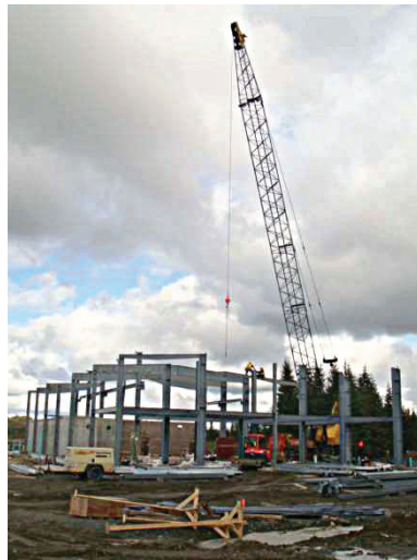
Significant work was completed on a new water treatment plant in 2008. Top left: The foundation concrete pour begins. Top right: The steel frame is erected. Bottom left: Interior view of state-of-the-art membrane water treatment equipment. Bottom right: Building exterior nears completion in December.
